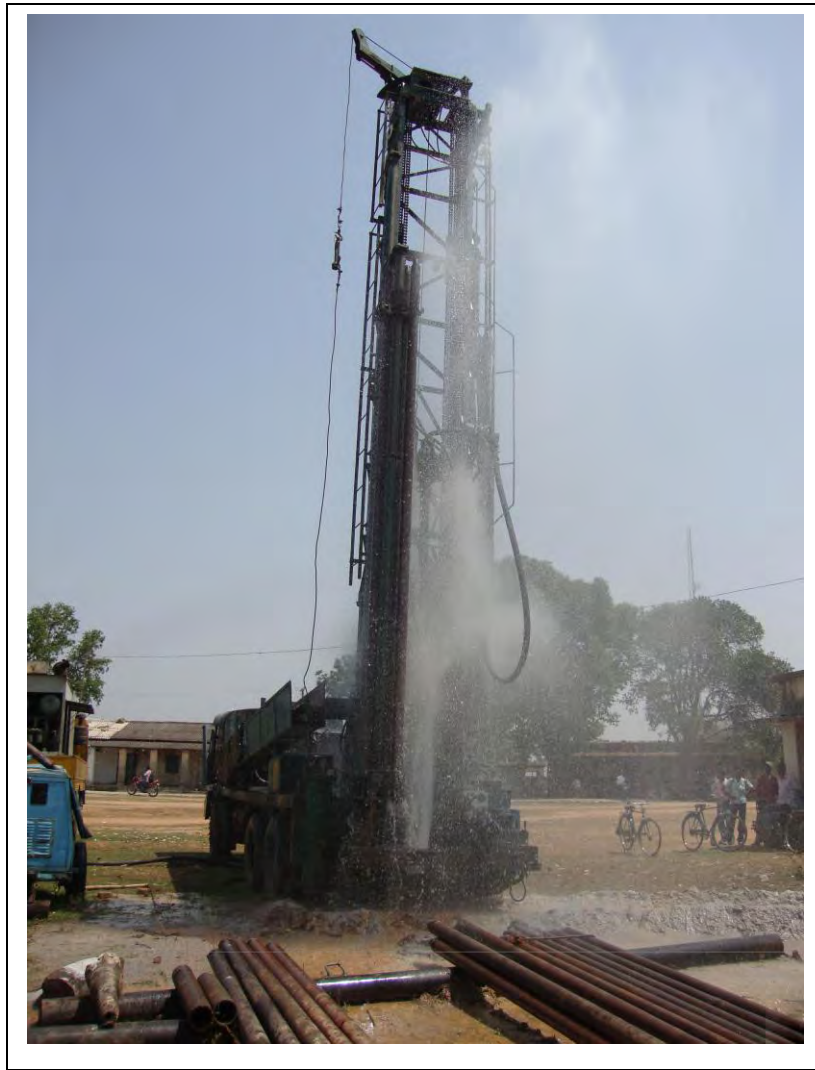
High yielding well at Karra, Khunti district (MER, Patna)
